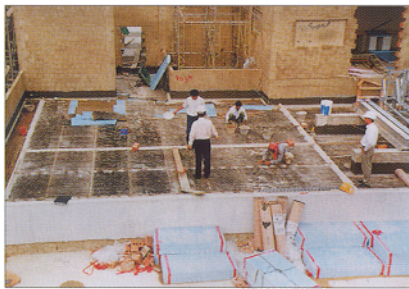
FIGURE 28 - LAYING OF INSULATION OVER RADCON #7
