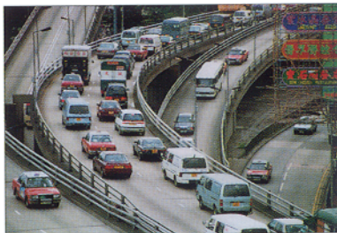
FIGURE 11 - CLOSE UP OF OVERPASS
