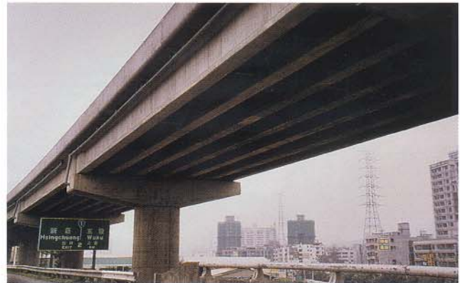
PHOTO 9 - UNDERSIDE OF RAISED FREEWAY
