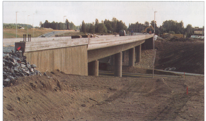
FIGURE 29 - KVERNDALEN BRIDGE, NOOSDLO
