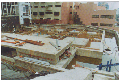
FIGURE 15 - ROOFTOP OF RETAIL LEVEL
