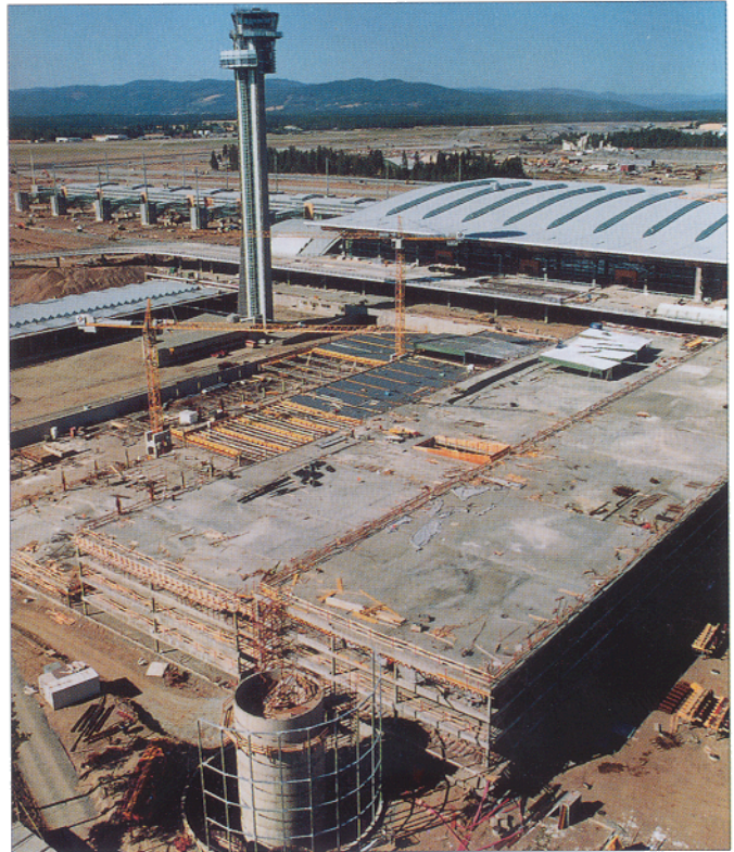
FIGURE 14 - GARDEMOEN AIRPORT UNDER CONSTRUCTION
