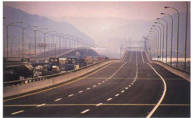
PHOTO 8 - FINISHED FREEWAY COVERED IN ASPHALT TOPPING
