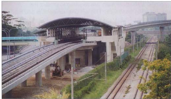
FIGURE 23 - LIGHT RAIL TRANSPORT STATION
