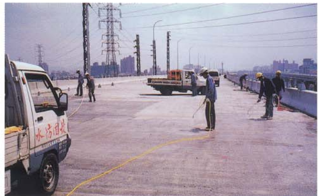
PHOTO 10 - RADCON #7 APPLICATION
