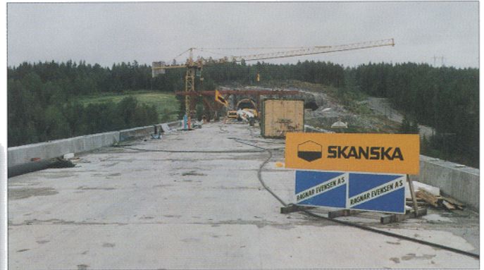
FIGURE 15 - BRIDGE DURING CONSTRUCTION
