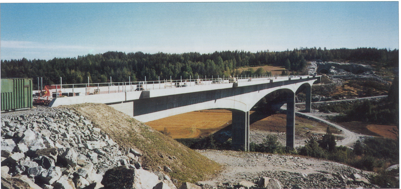
FIGURE 14 - HOLENDALEN RAILWAY BRIDGE, NORWAY
