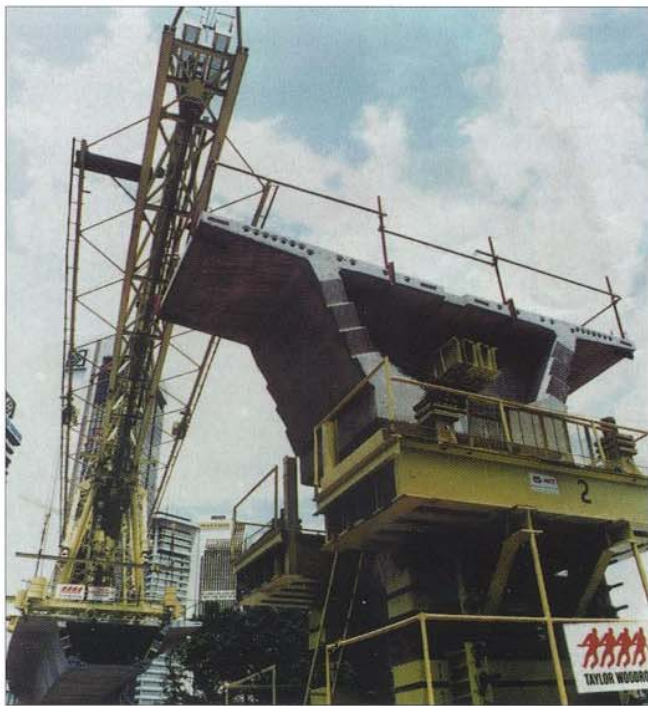
FIGURE 21 - GANTRY TRANSPORTED FROM AUSTRALIA TO MALAYSIA
