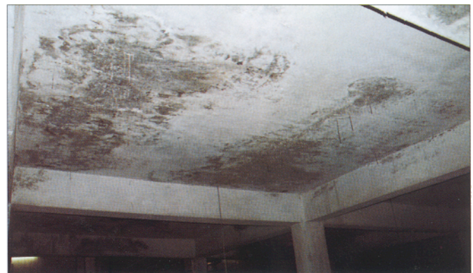
FIGURE 31 - SOFFIT WITH 300MM CALCIUM STALICTITES
