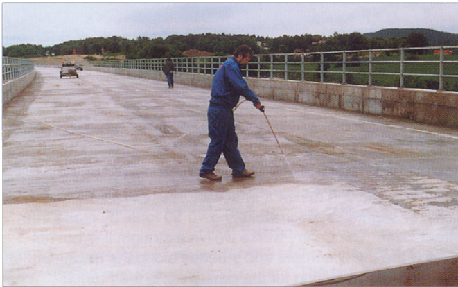
FIGURE 24 - RADCON #7 APPLICATION
