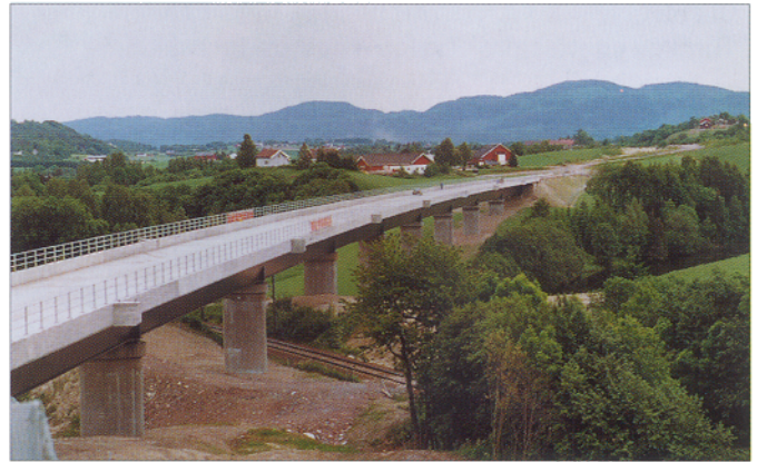
FIGURE 25 - BREMSA BRIDGE, NORWAY
