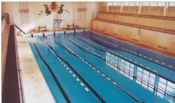
FIGURE 30 - SWIMMING POOL RE-FILLED AFTER SUCCESSFUL REPAIRS
